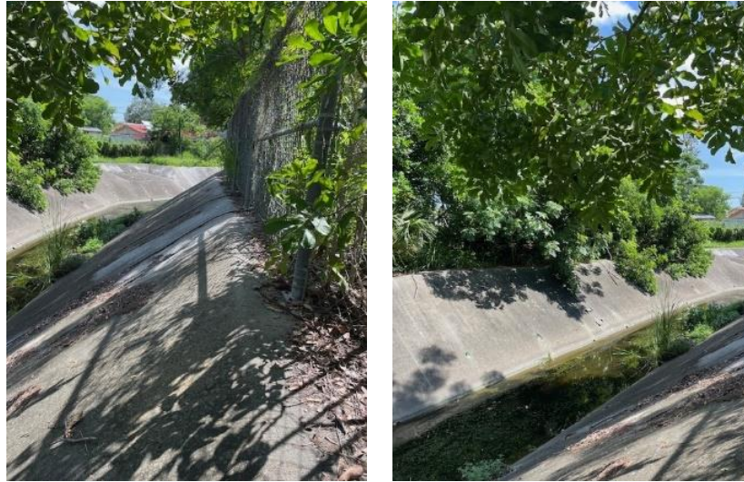
Photos 1 & 2: Concrete swale showing invasive vegetation on far side (inaccessible) and additional views of the concrete swale illustrating its depth and steep slope.
