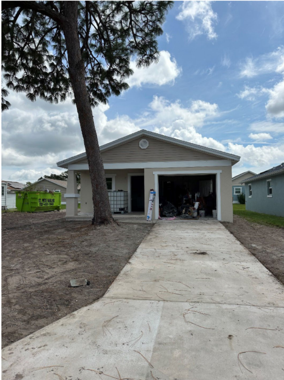
Site Photo at 6243 67 th Lane N.
